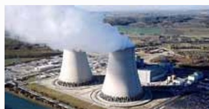
EDF nuclear power station
